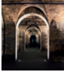
Chq-building Dublin (Ireland)
