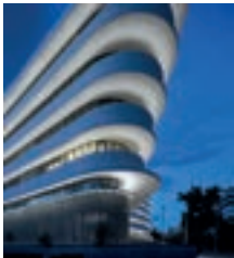
Agemar HQ Athens (Greece) Project: Arch. Eleftheria Deko Photography: Nikos Daniilidis
