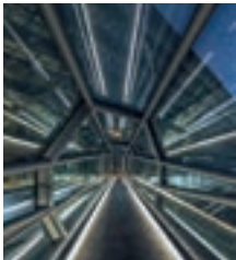
Capricorn Bridge Dusseldorf (Germany) Project: Arch. SUPERGELB Architekten Photography: HGESch
